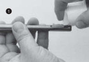
Fig. 1: Cleaning of connection ends
